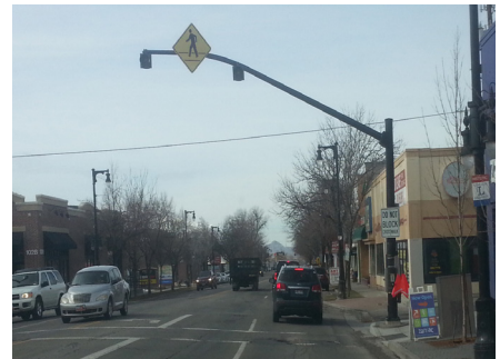
Figure 1 - Overhead Flashing Beacon
